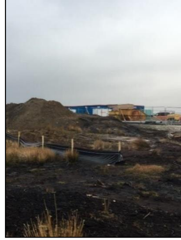
Figure 5 Typical Silt Fences used on Oweninny Wind Farm Phase 1
