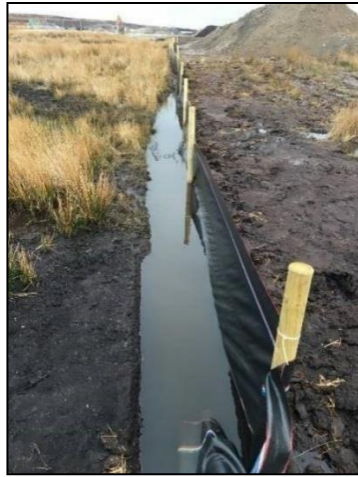
Figure 5 Typical Silt Fences used on Oweninny Wind Farm Phase 1
