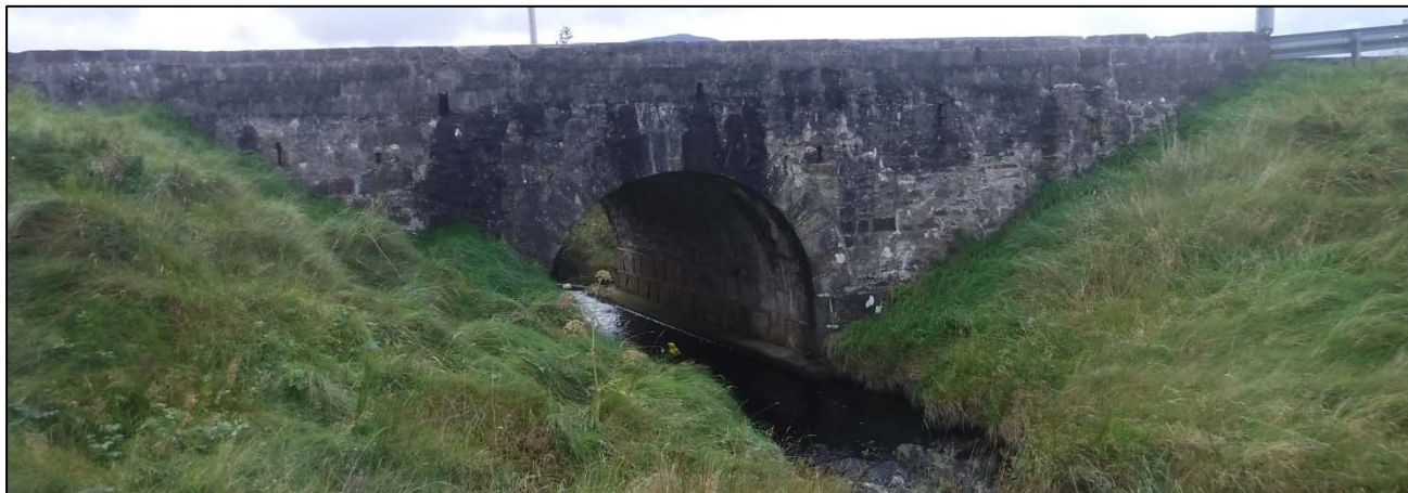
Plate 3 The Western Way Bridge – Upstream View
